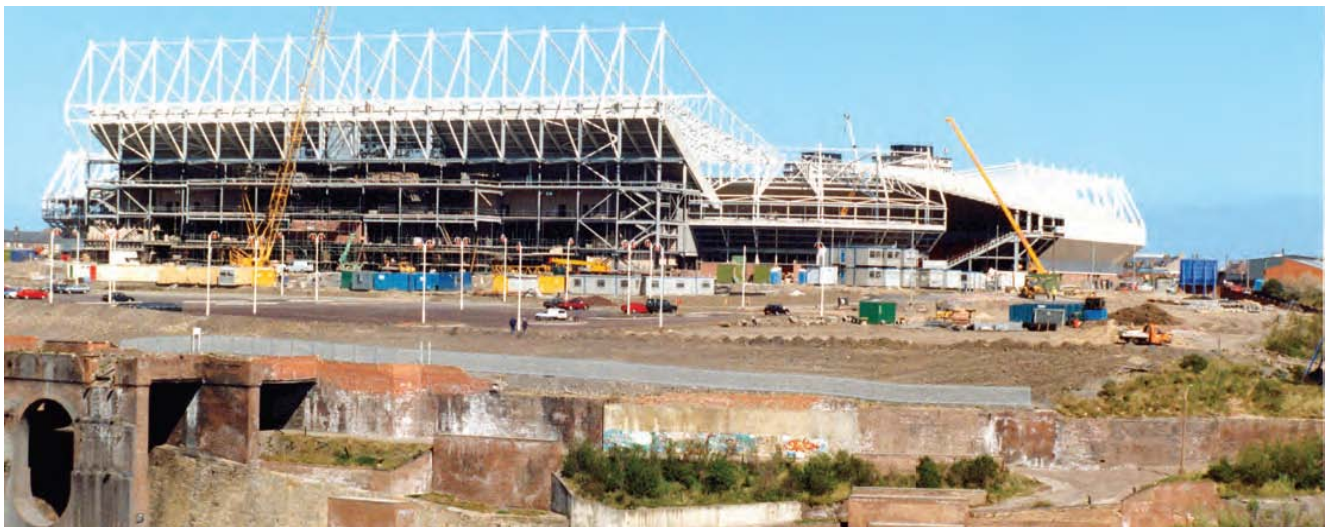
Picture: Building Sunderland Football Club's Stadium of Light 1997
